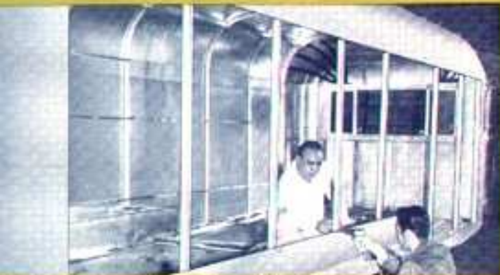
The ribs are placed in position and the sides are being riveted on.
