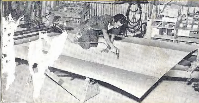
Silver Streak's chassis is wrapped with spun glass insulation. Note that the chassis is completely covered with aluminum.
