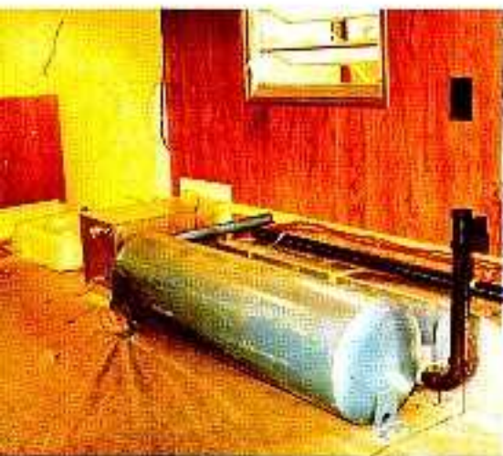
All plumbing located above floor for positive drainage, protection against road hazards and the outside elements
