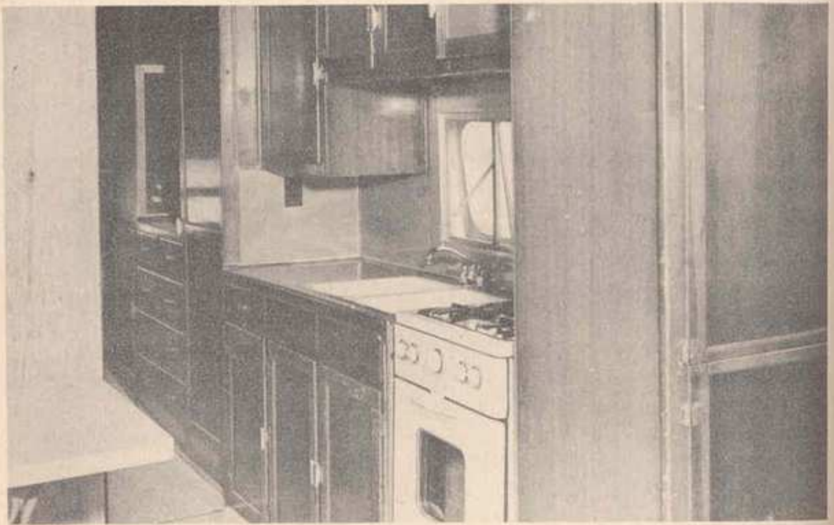
Picture 8. Old ice box is replaced by new stove. Old sink is replaced with new double sink and swing faucet. Sink drainboard is recovered with Formica.
