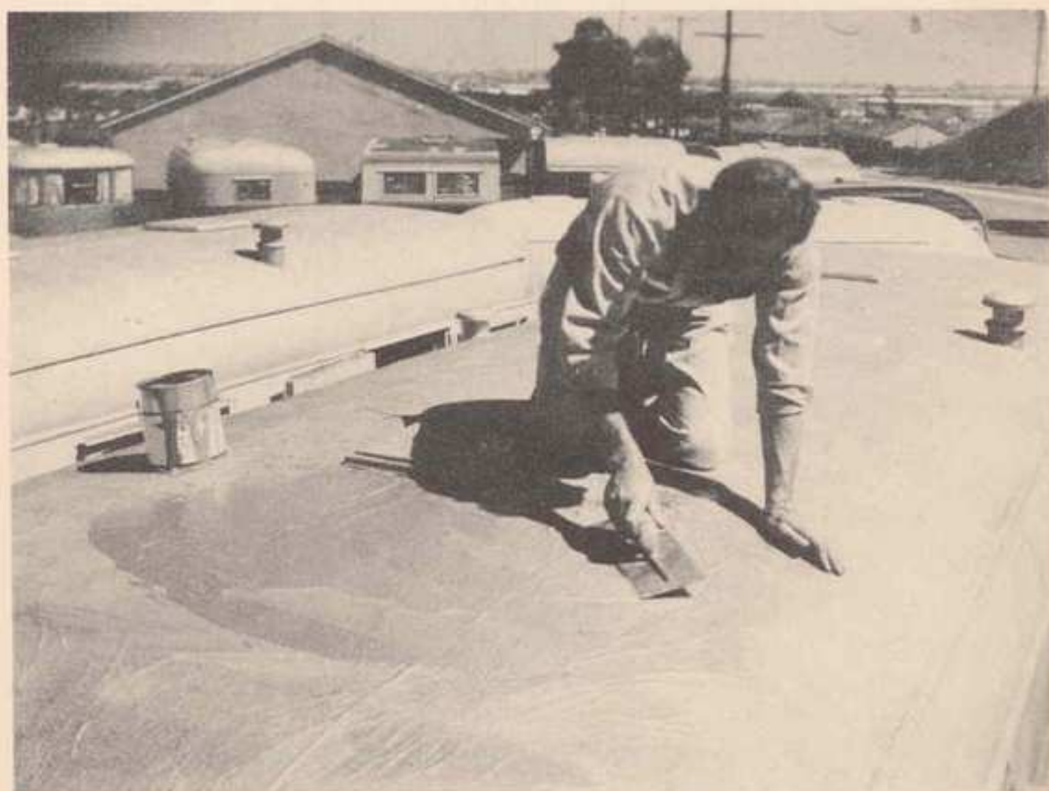
Pictures above show easiest method for applying roof mastics.
